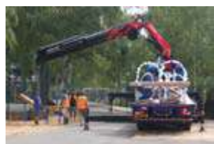
Site installation Summer 2020
