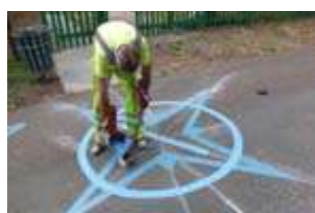
Test Panel September 2020
