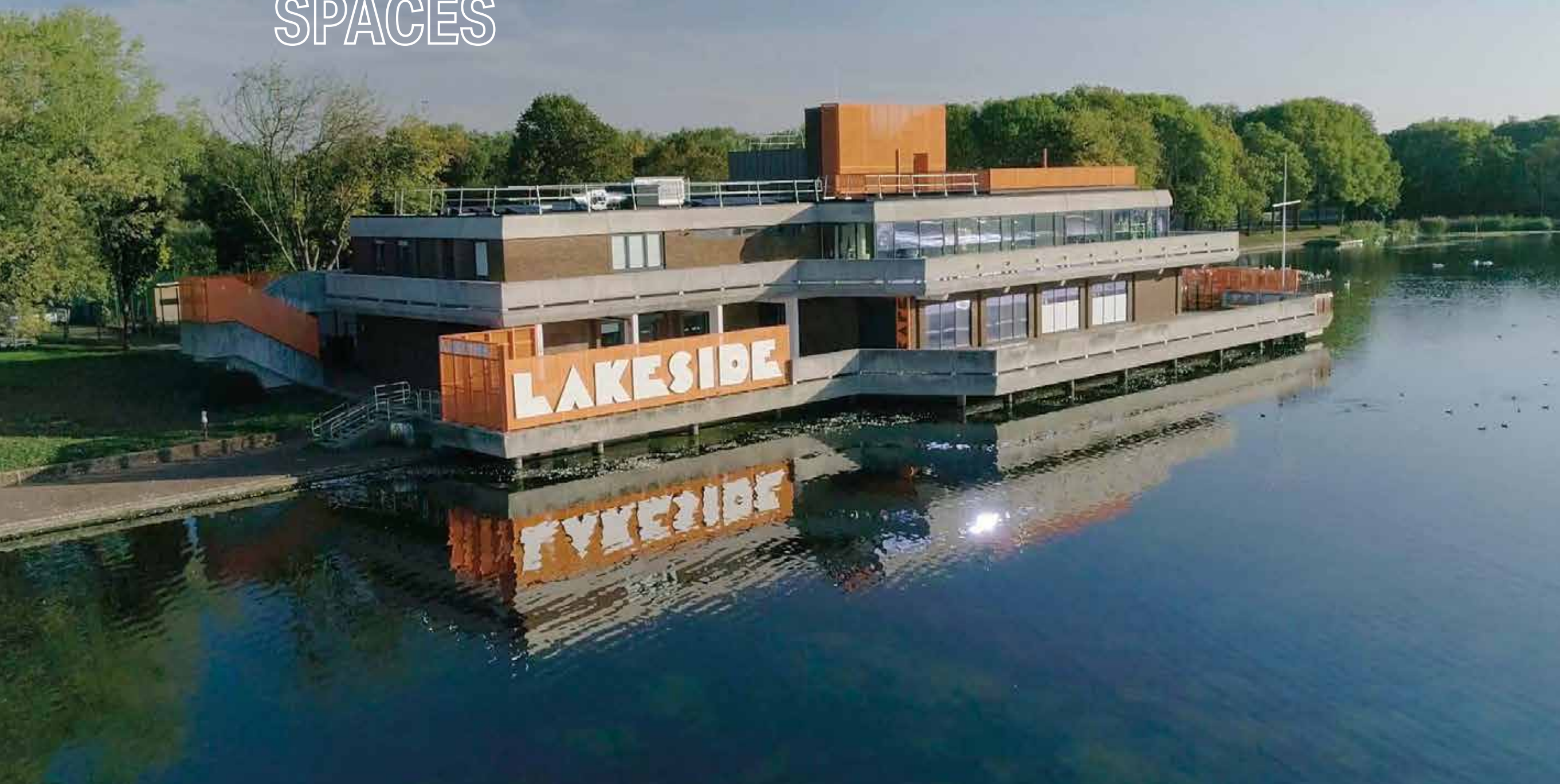
Renovation of Lakeside Centre completed in 2019 by Bow Arts with support from the Mayor of London and the London Economic Action Partnership (LEAP), Peabody and Arts Council England.
